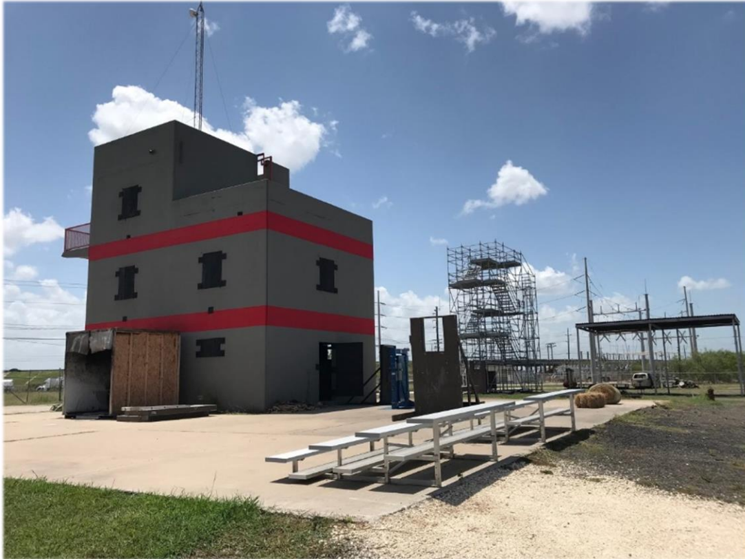
FIGURE 2-10: BFD Training Facility
