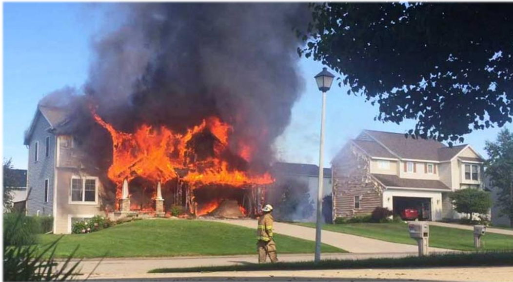
FIGURE 2-5: Fire in a Residence that was not Equipped with Residential Sprinklers
