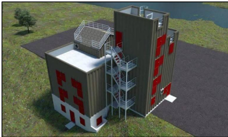
FIGURE 2-20: Typical Fire Training Tower and Burn Building
